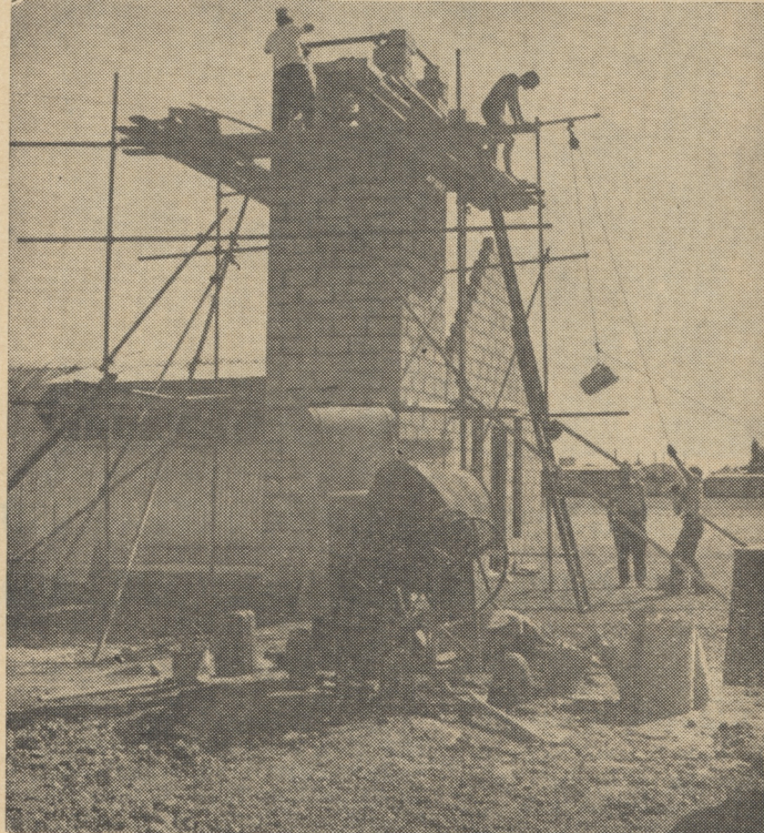
These "during and after" pictures (see right) indicate the amount of work that was required to make the chapel in Camp Maple Leaf a fit place for worship. Under the direction of Father Romeo Plourde this and considerable interior renovations were made.
